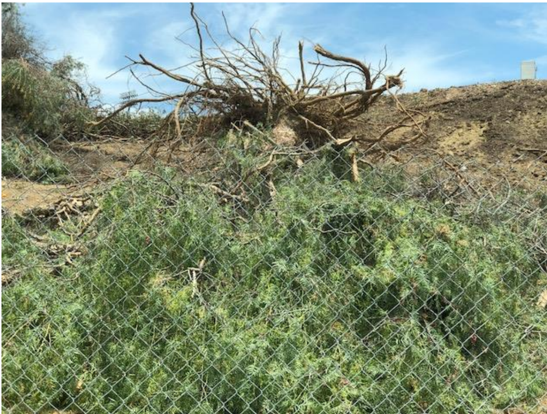
Clear and Grub (Landscape Removal)
