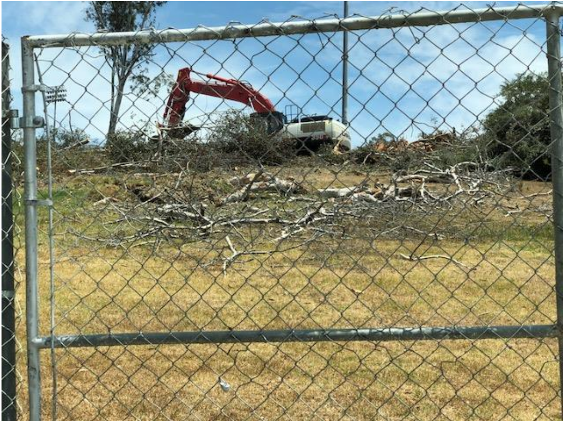
Landscape Removal around Stadium Facility
