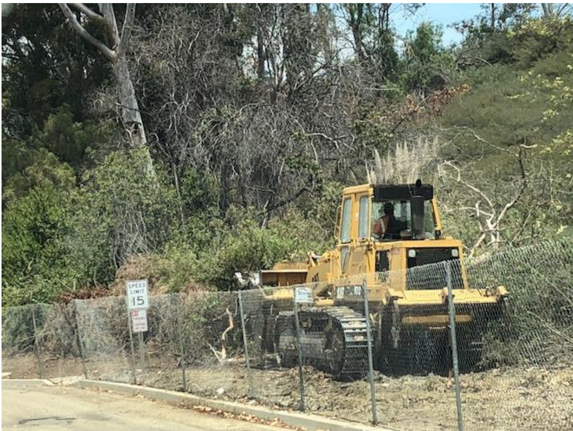
Landscape Removal around Stadium Facility
